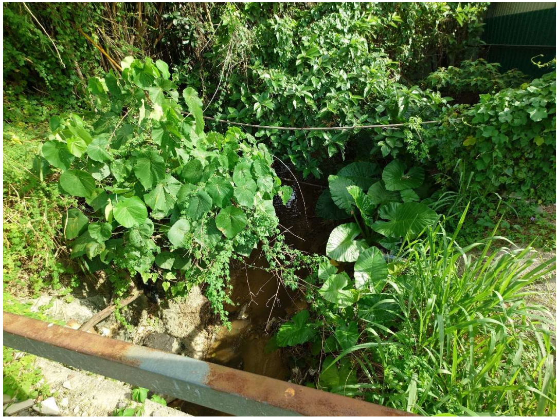
Photo for Existing Open Stream Course
